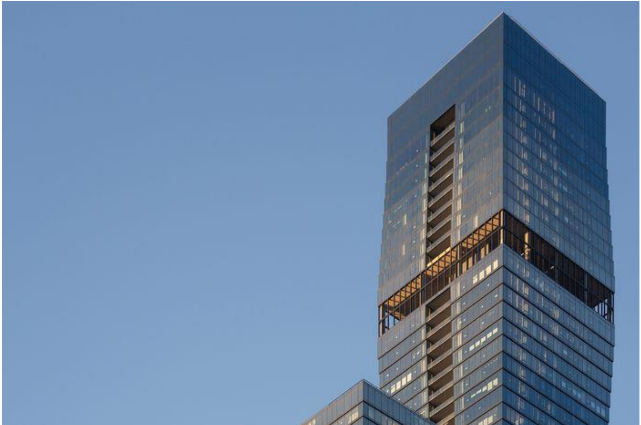
View of the 'blow through' at the St. Regis | PHOTO: ANGIE MCMONIGAL/STUDIO GANG
